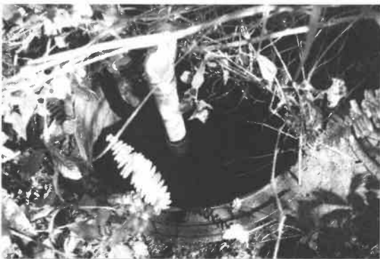
Package wastewater treatment plant well.
