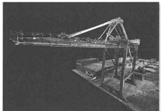
CB&I laser scan of the Port Charleston
