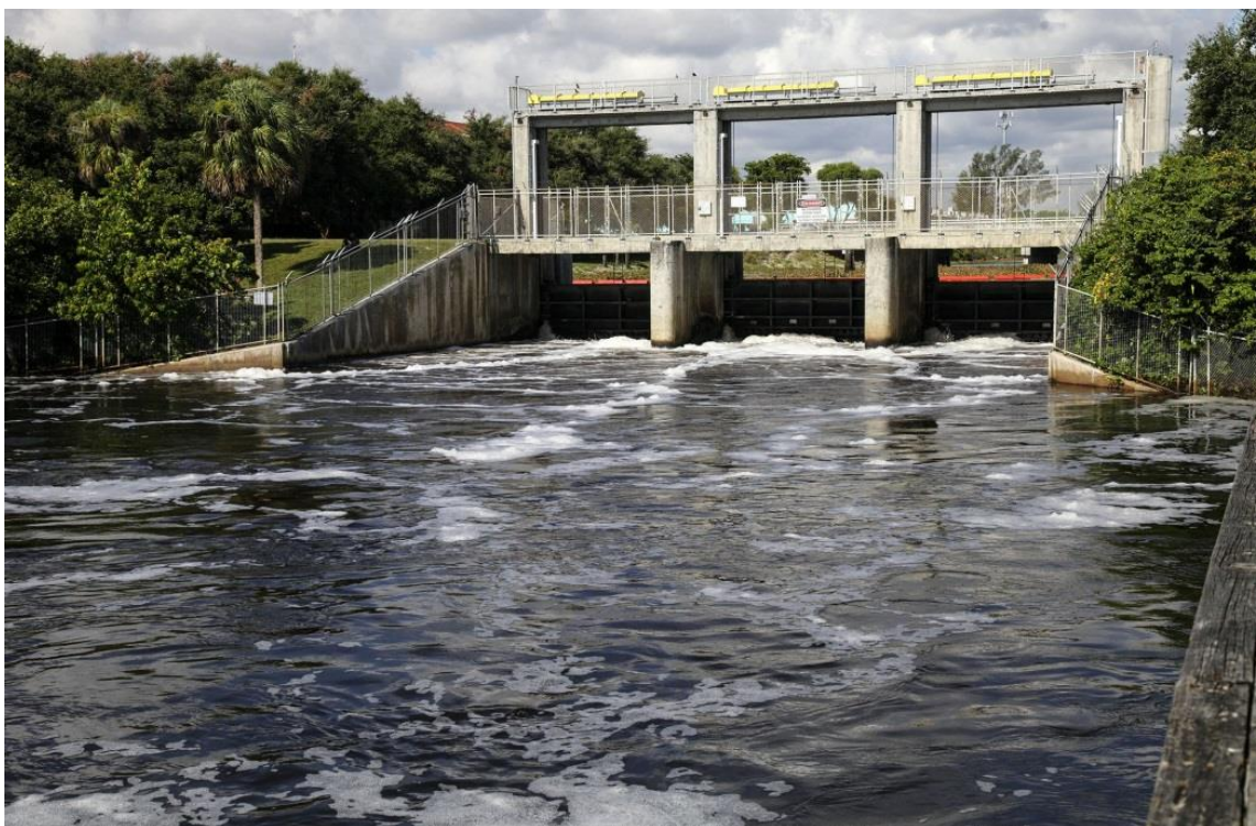
Figure 2: SFWMD Flood Control Structure, Boynton Spillway
