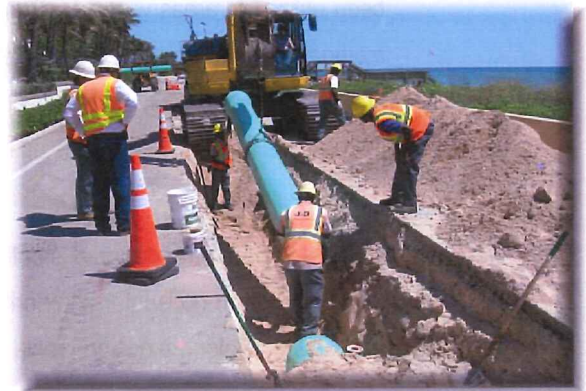
Force Main Replacement
