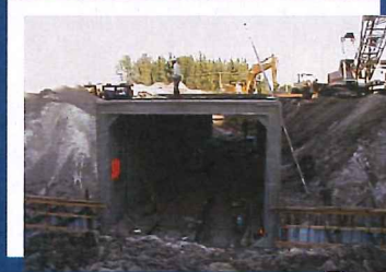
Client: City of Delray Beach Project: L-33 Canal Culvert
