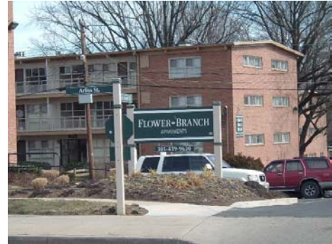
The panel recommends that the County consider the future of the Flower Branch Apartments.
