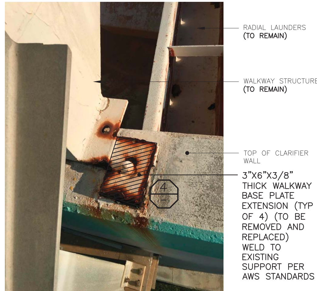
EXISTING WALKWAY STRUCTURE CONNECTION TO CONCRETE TANK N.T.S.
