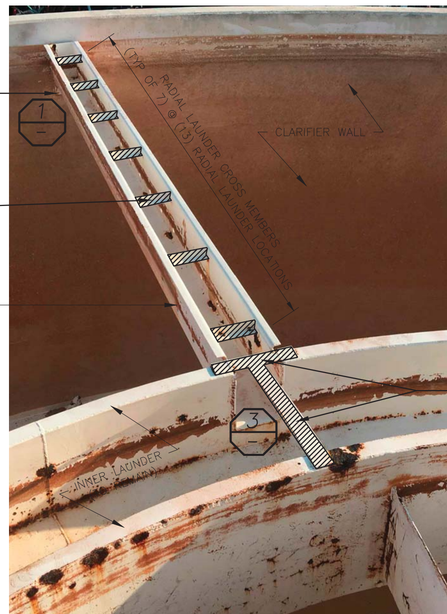
EXISTING EFFLUENT LAUNDERS AND "T" SUPPORTS N.T.S.
