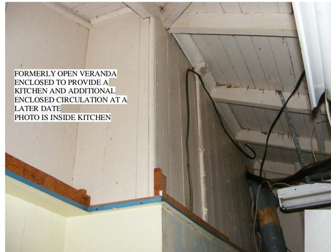
FORMERLY OPEN VERANDA ENCLOSED TO PROVIDE A KITCHEN AND ADDITIONAL ENCLOSED CIRCULATION AT A LATER DATE
