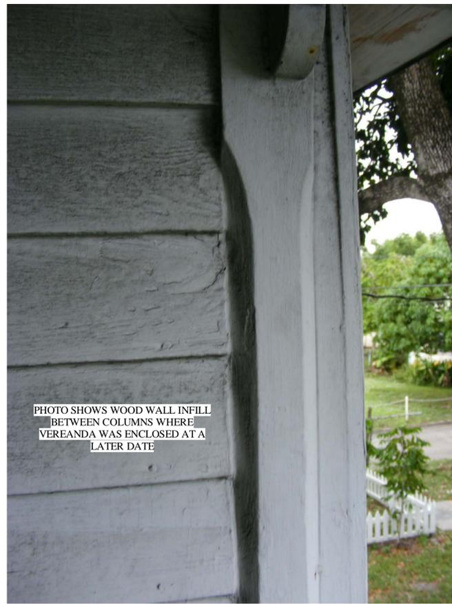
PHOTO SHOWS WOOD WALL INFILL BETWEEN COLUMNS WHERE VEREANDA WAS ENCLOSED AT A LATER DATE
