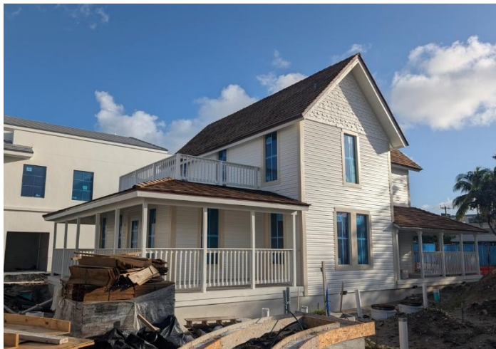
Existing rear (west) elevation of Building A (The Rectory)
