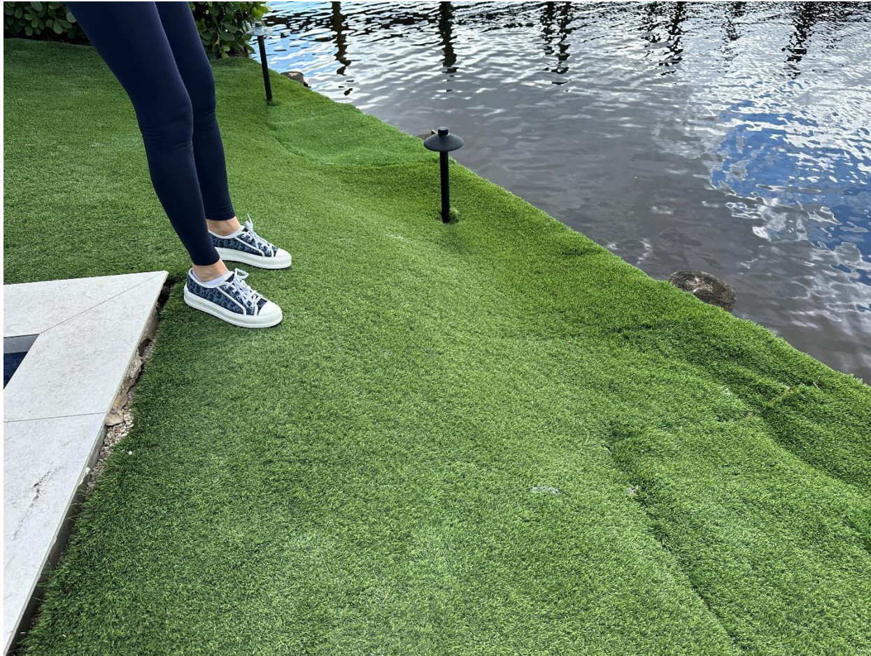
SOUTH END SINKHOLES STEEP SLOPE, Failing at pool coping.
