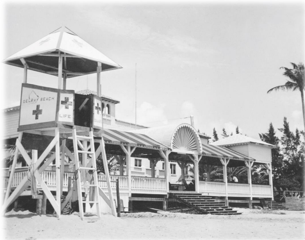
FIGURE 18. The Pavilion and Lifeguard Station at the end of Atlantic Avenue.
