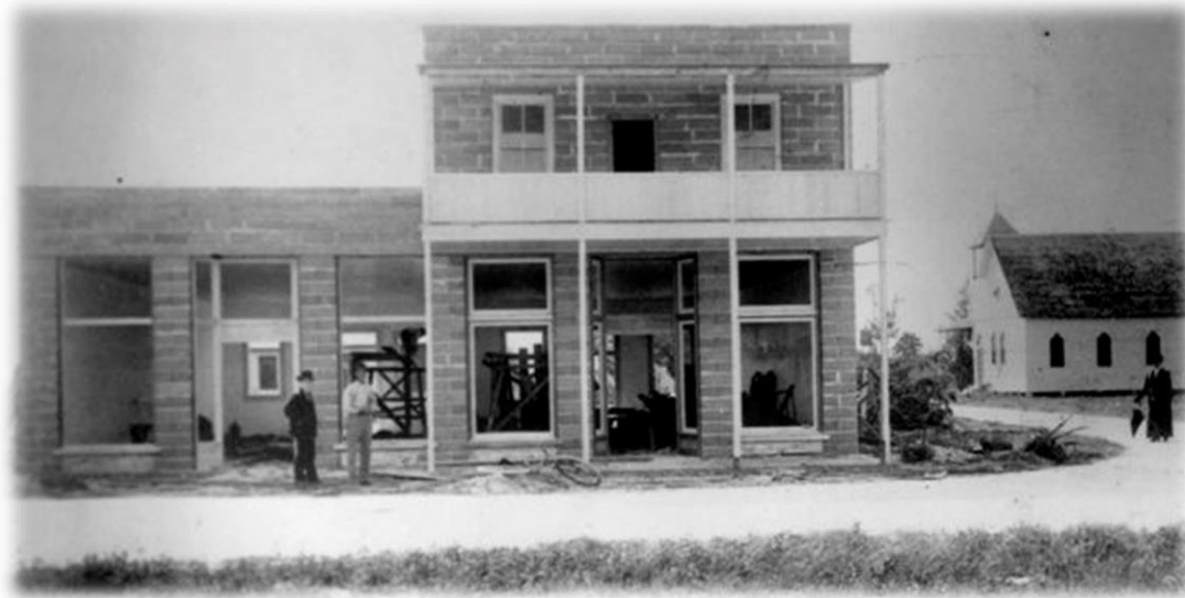
2-4 East Atlantic Avenue during construction Source: City of Delray Beach Historic Preservation Office
