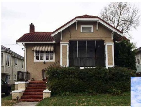
(a) Photo: Rubion Construction Co., LLC
