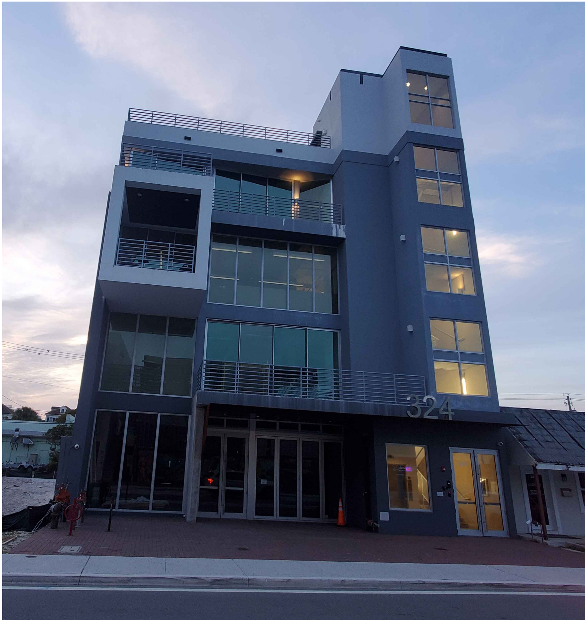
EXIST. BLDG. PHOTOGRAPH A
