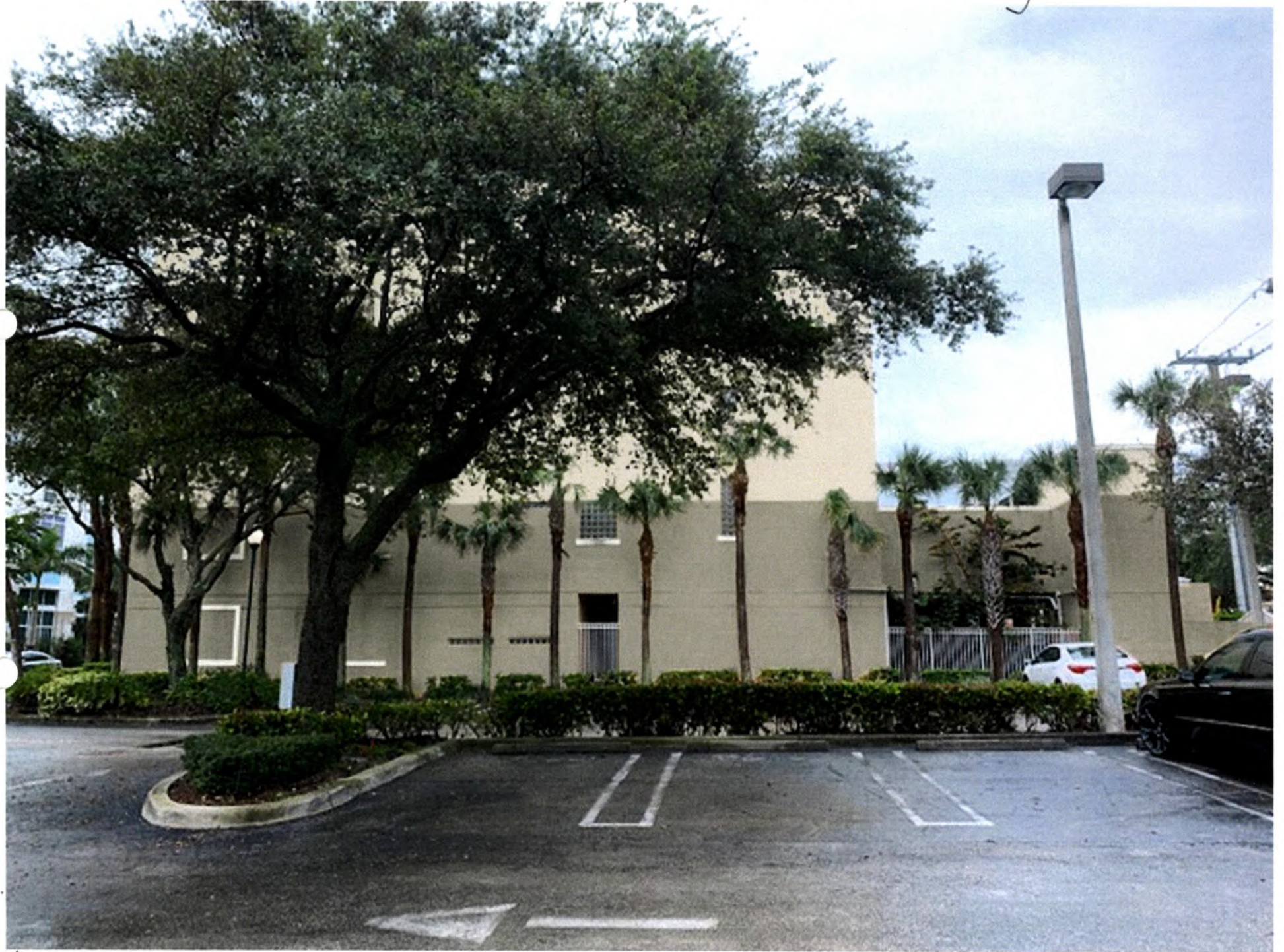
New Paint North Side of Bldg
