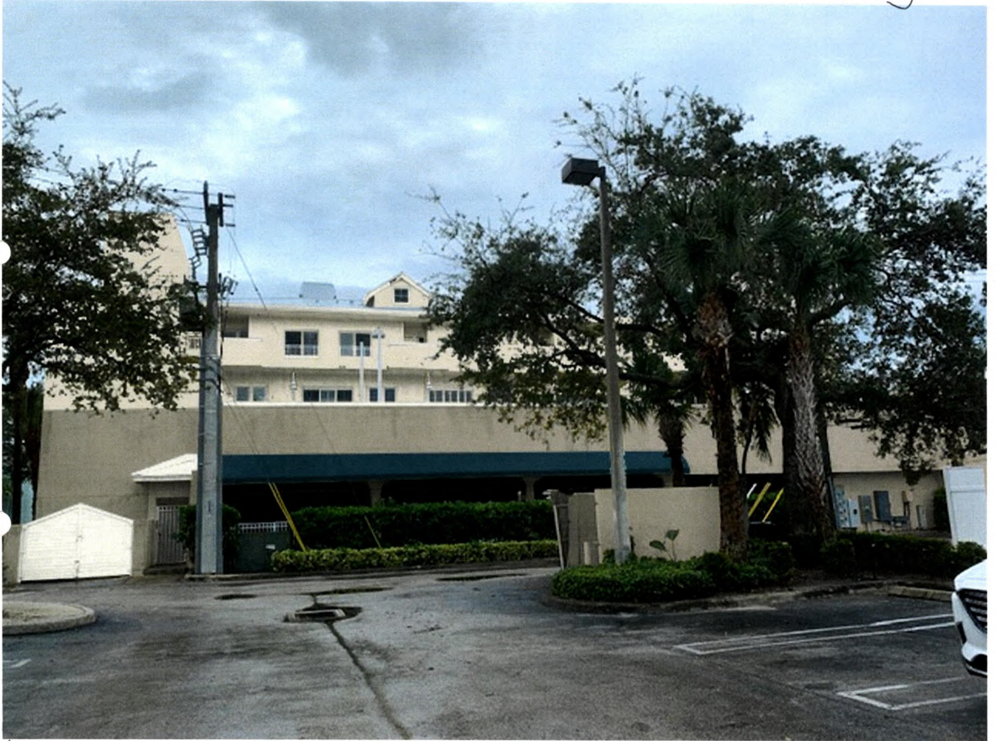
New Color on West Side of Bldg
