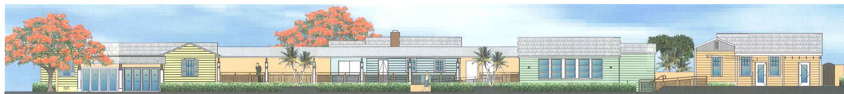
East Elevation (Facing Pool-Not Visible from Street)
