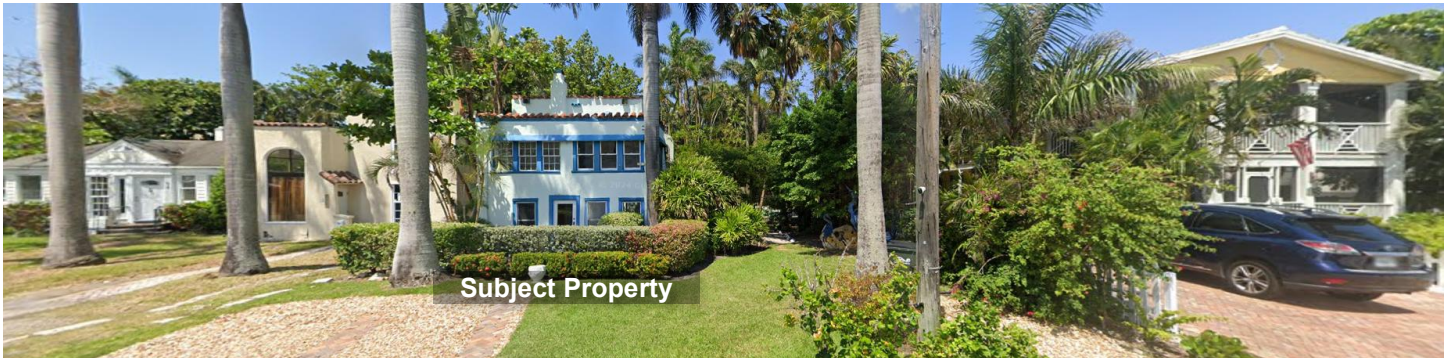
Existing streetview - Marine Way
