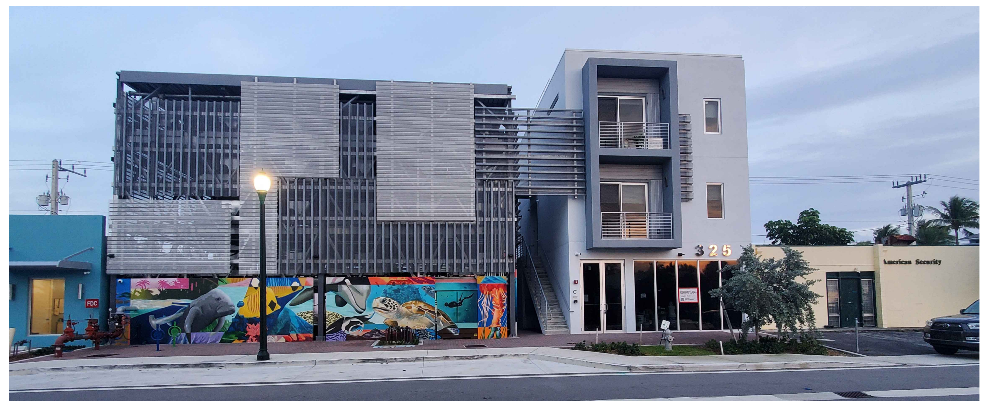
EXIST. BLDG. PHOTOGRAPH C SCALE N.T.S.
