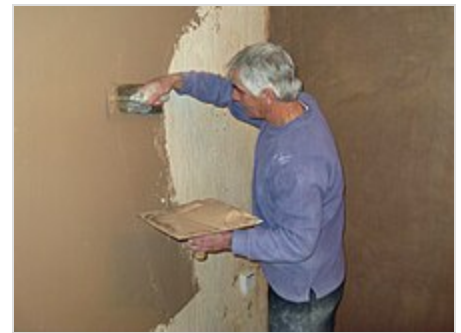
Plastering an internal wall
