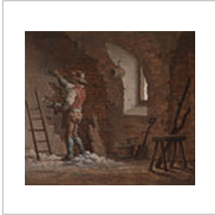
Early 19th Century plasterer at work – painting by John Cranch (1751–1821)
