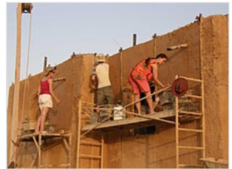
Applying mud plaster to an outside wall
