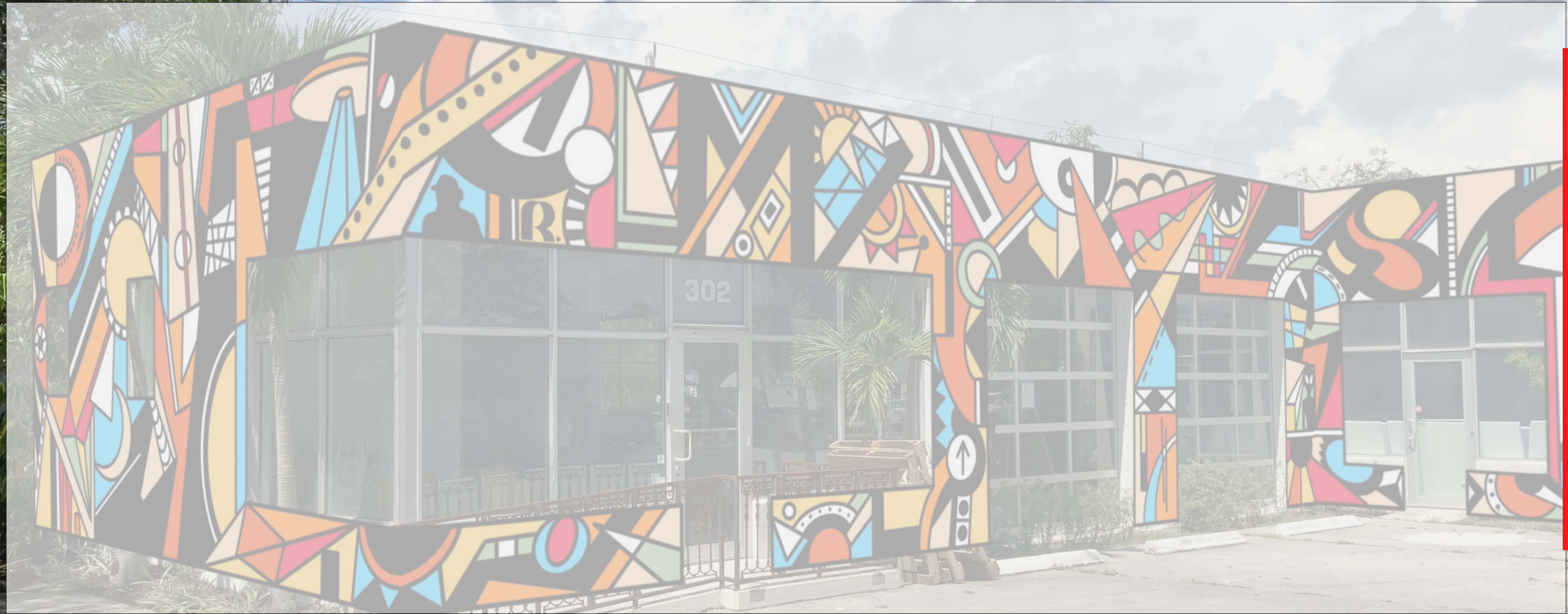
Exterior Latex Paint and UV Protective Clear Coat on top.
