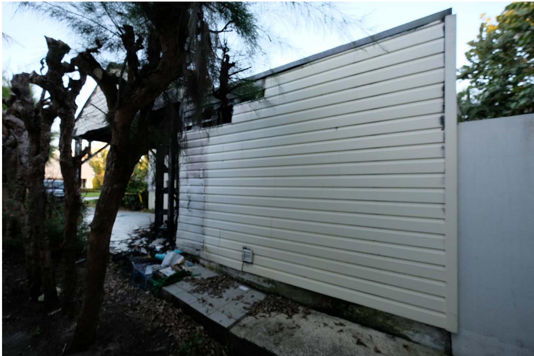
1120 NASSAU STREET - WEST FACADE
