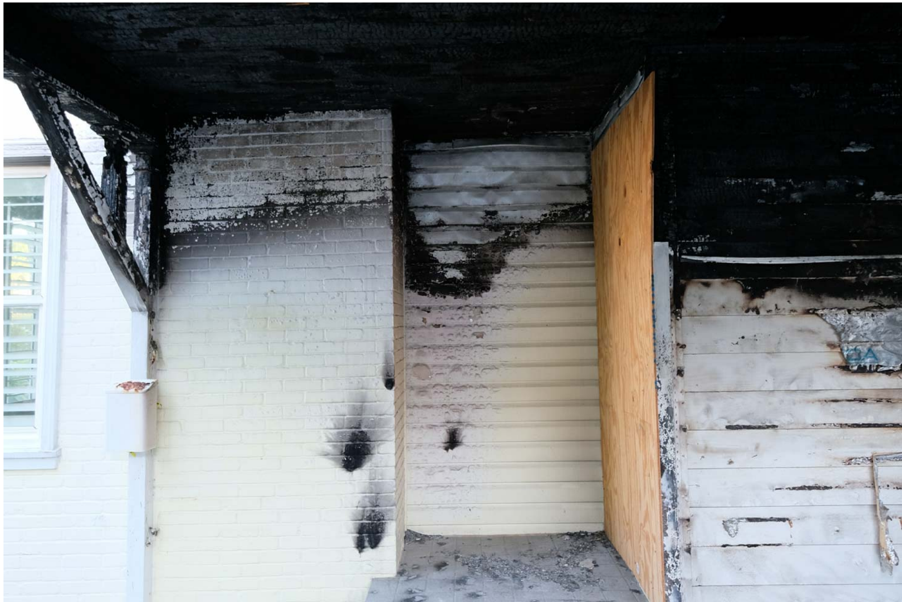
1120 NASSAU STREET - WEST FACADE
