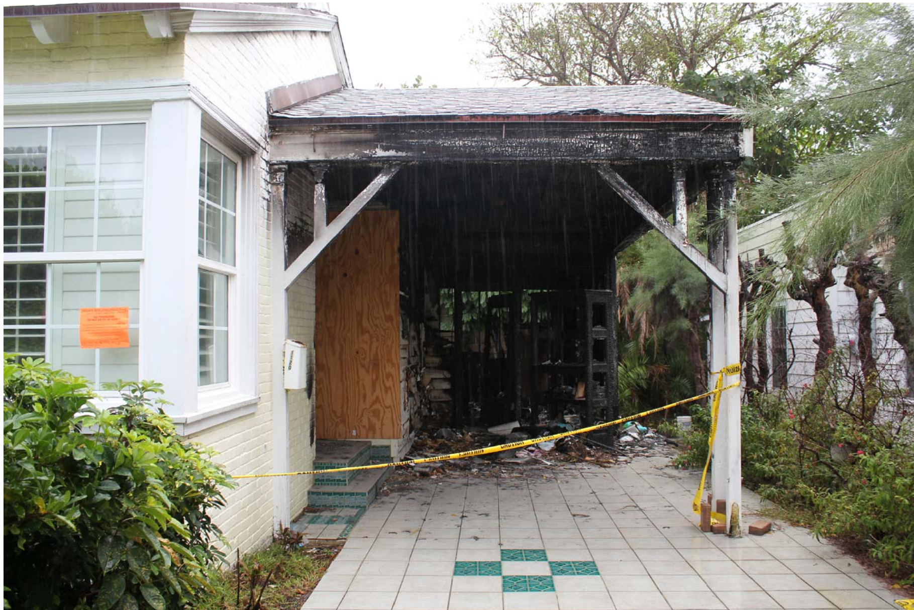
1120 NASSAU STREET - NORTH FACADE
