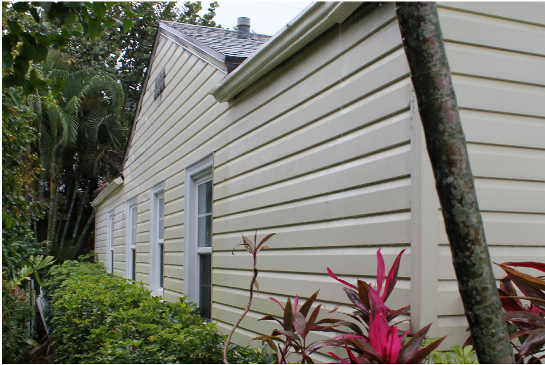
1120 NASSAU STREET - EAST FACADE
