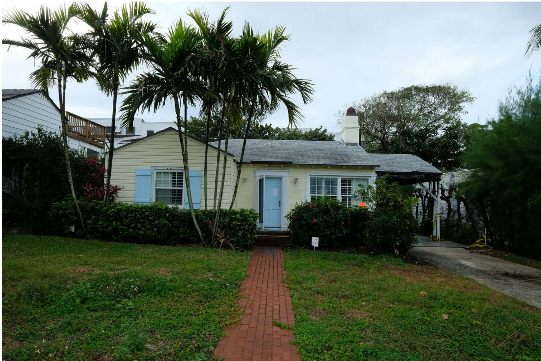
1120 NASSAU STREET - NORTH FACADE
