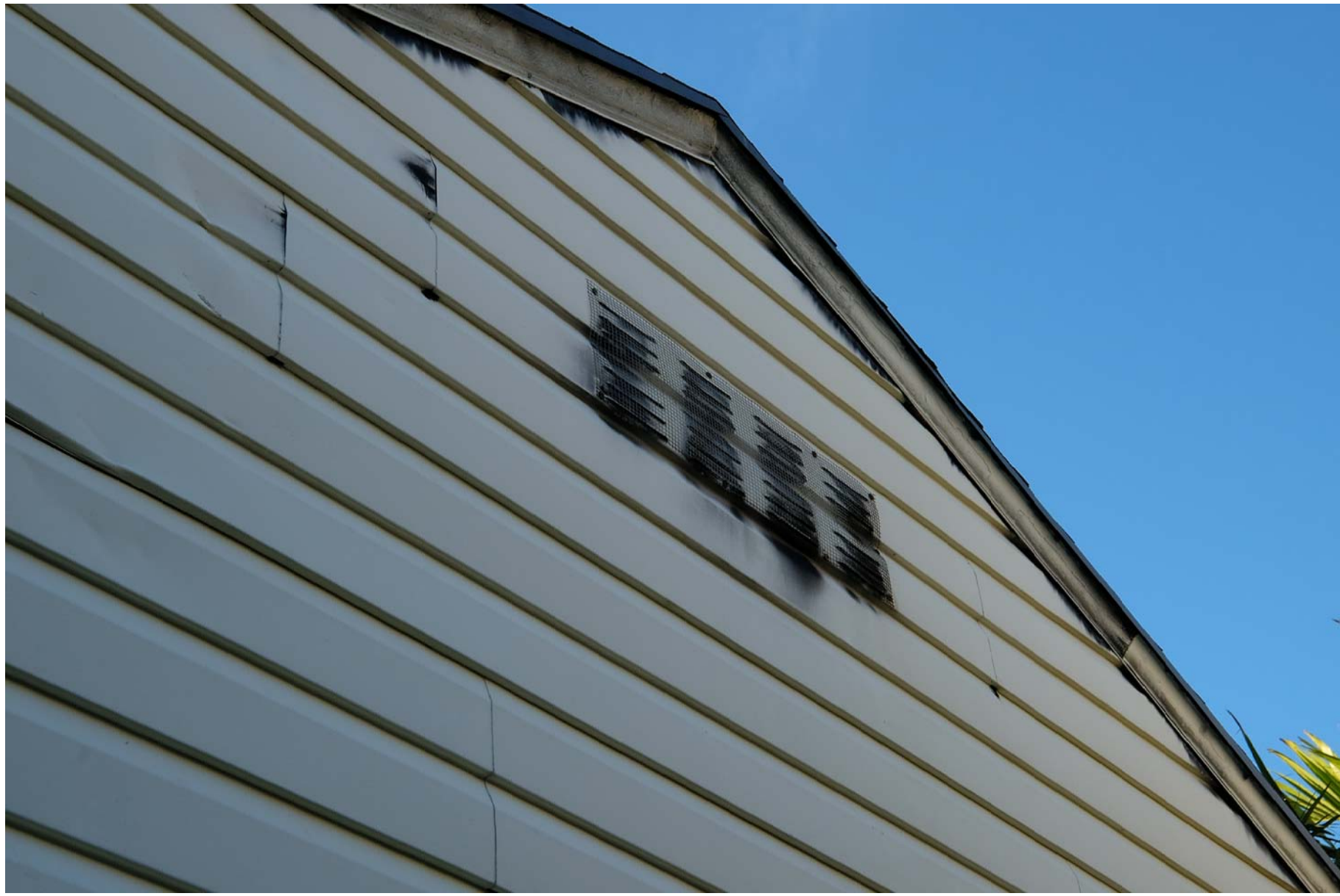
1120 NASSAU STREET - EAST FACADE
