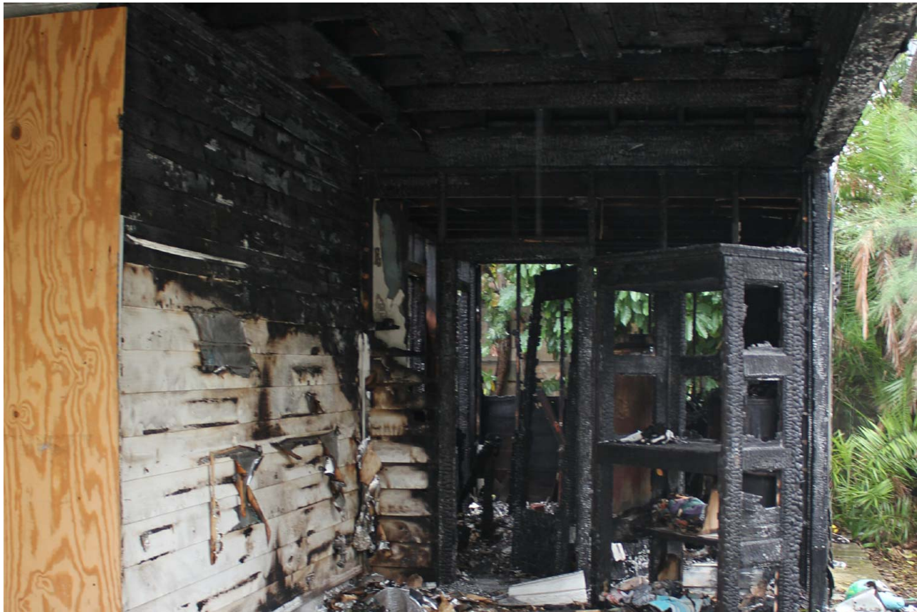
1120 NASSAU STREET - NORTH FACADE
