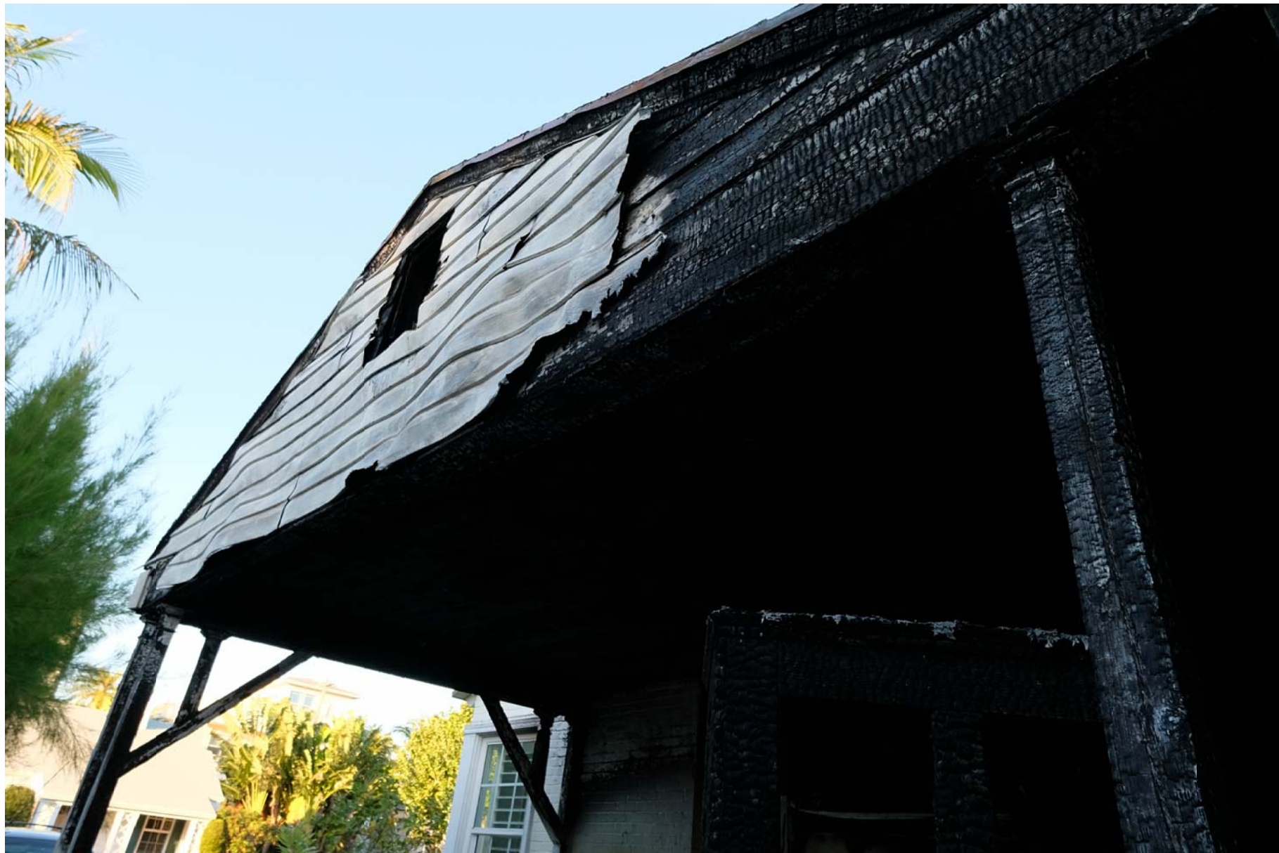
1120 NASSAU STREET - WEST FACADE
