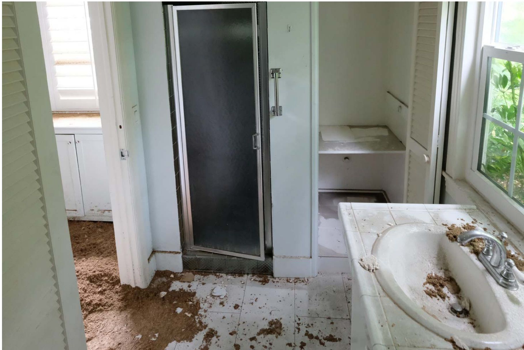
1120 NASSAU STREET - BATHROOM
