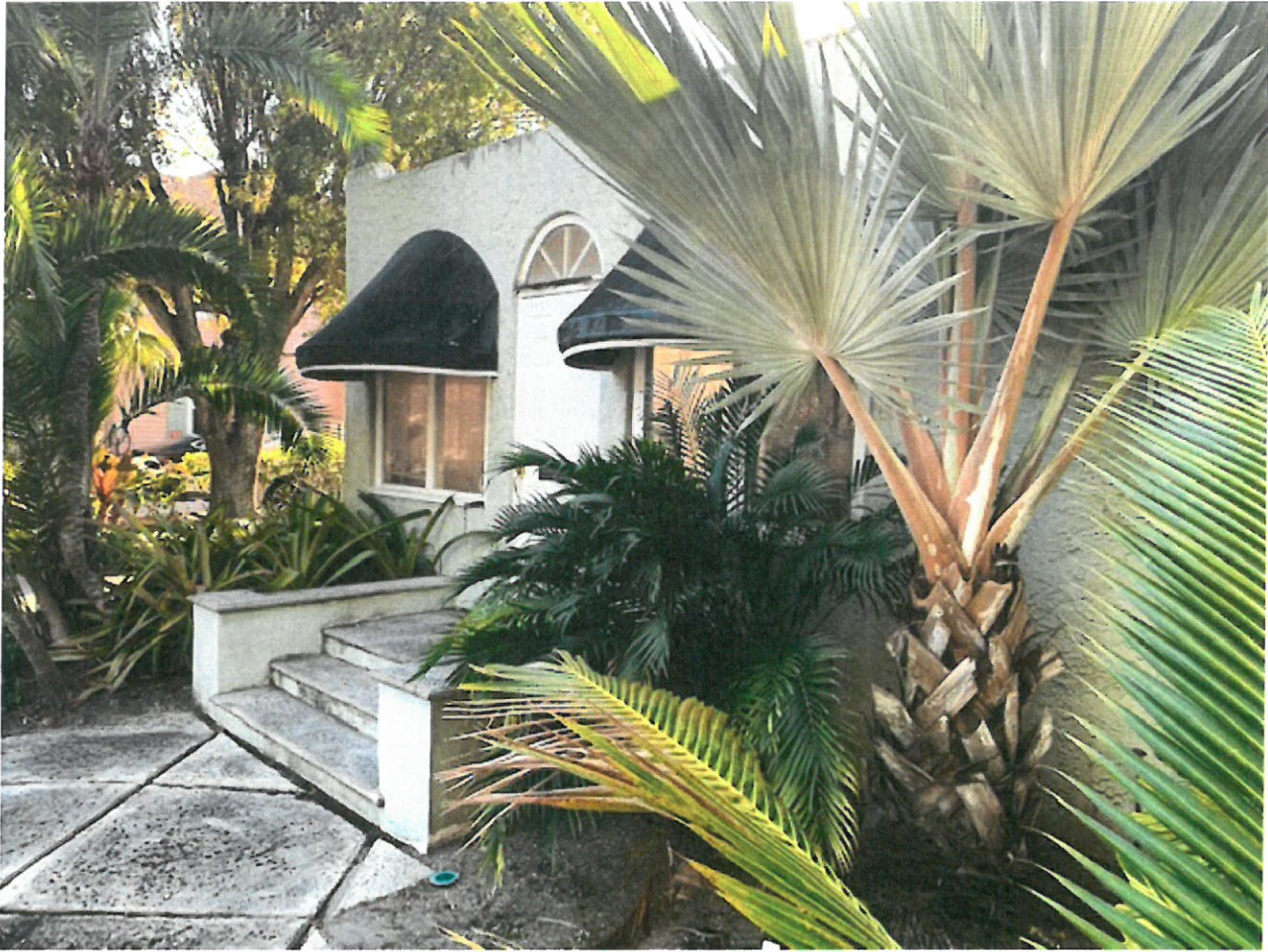
East Elevation - Main Building
