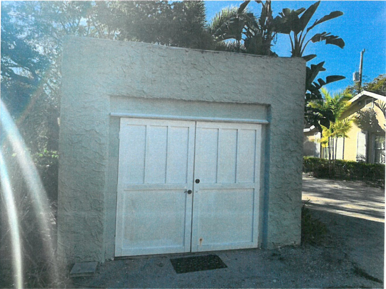
East Elevation - Storage Building
