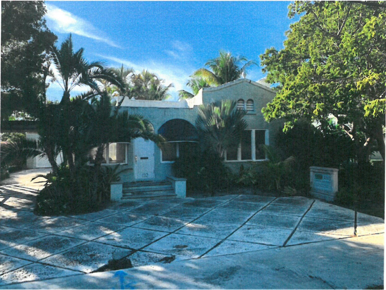
East Elevation - Main Building
