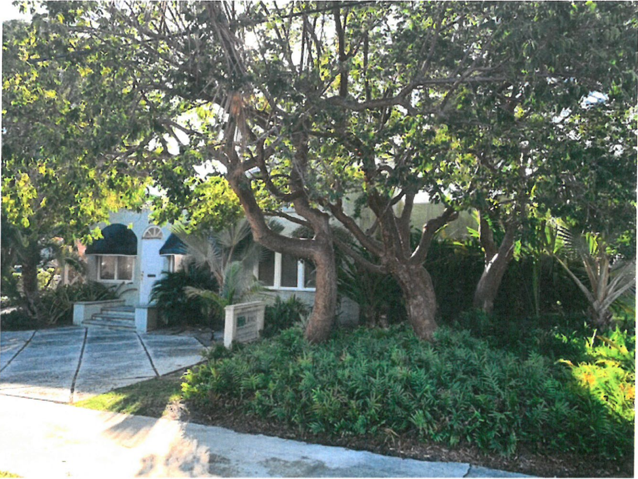
East Elevation - Main Building
