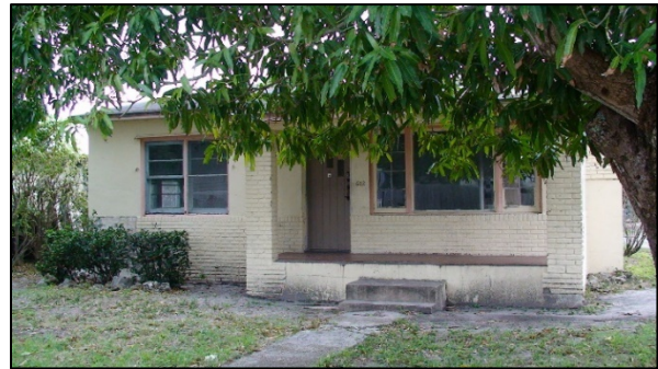
Abandoned Home in Delray Beach
