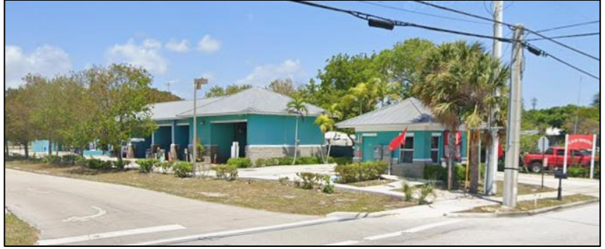
Existing Car Wash
