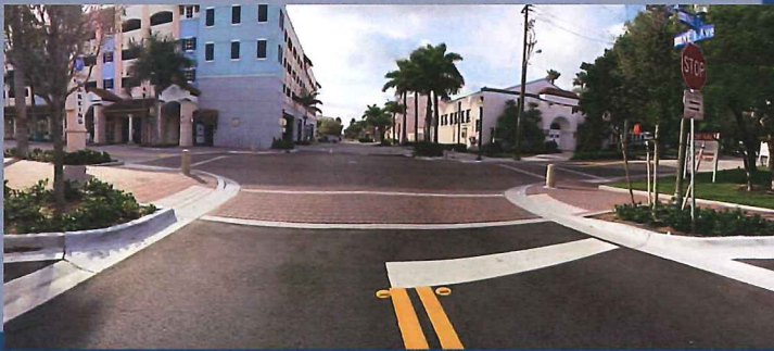
Client: City of Delray Beach Project: NE 1 st Avenue Improvements
