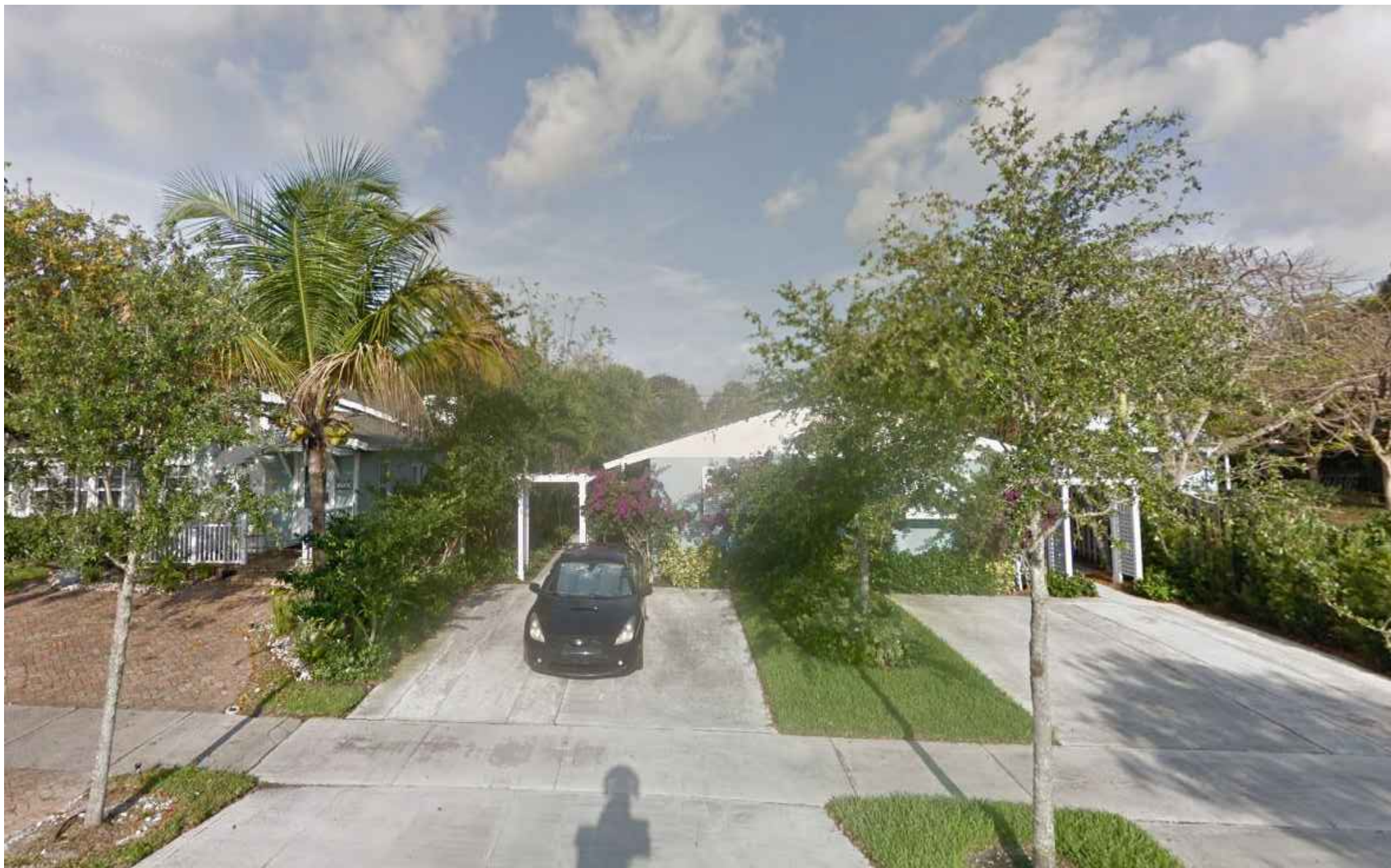
EAST ELEVATION-320 NE 1ST AVE
