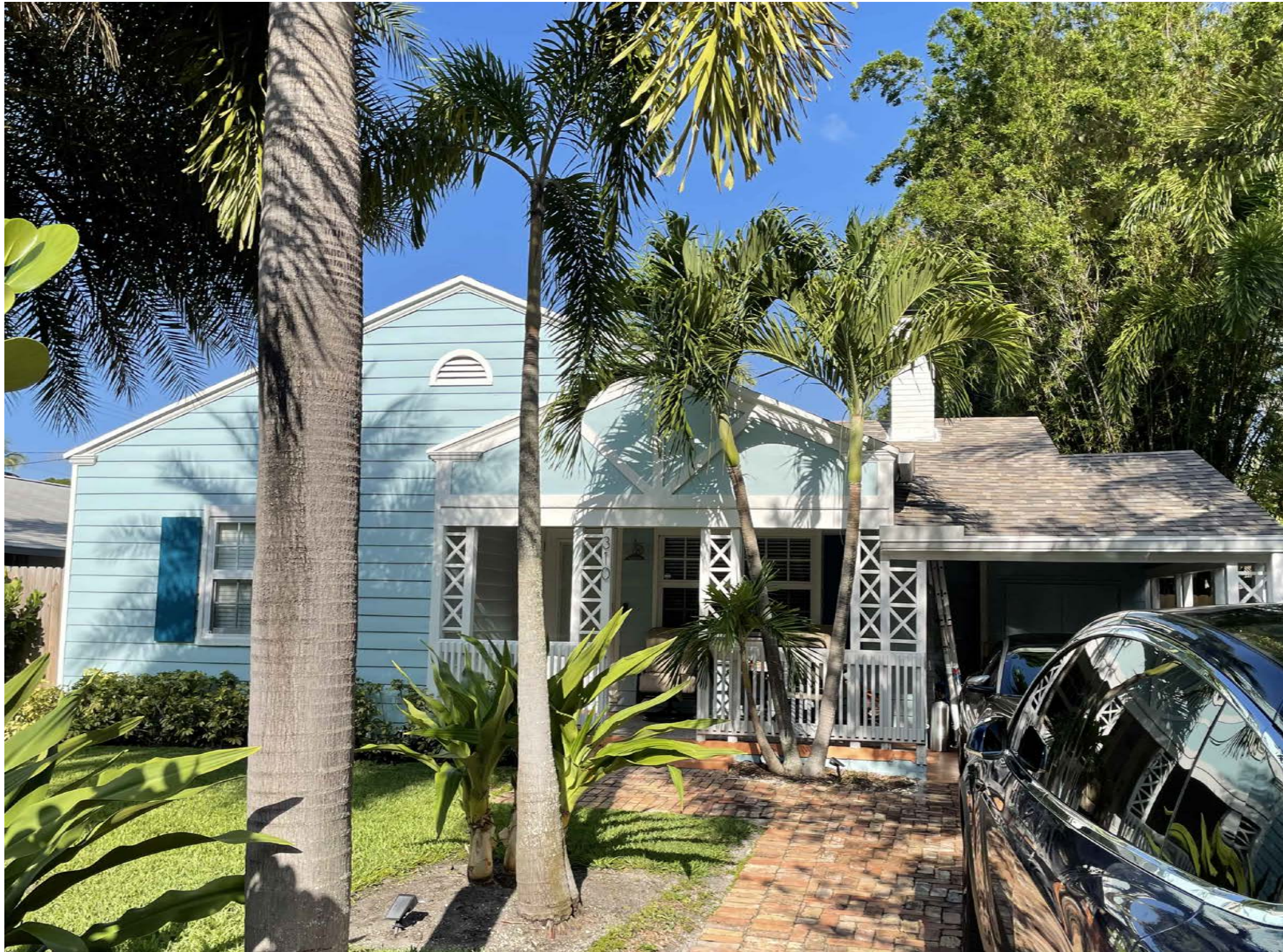
EAST ELEVATION-310 NE 1ST AVE
