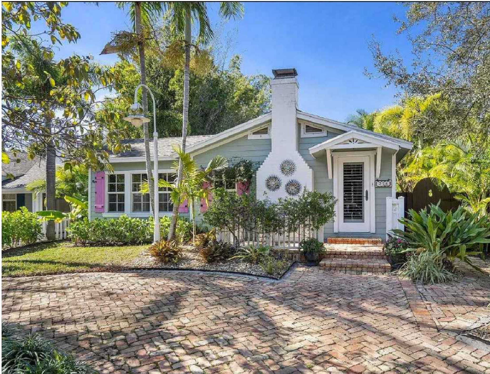
EAST ELEVATION-314 NE 1ST AVE
