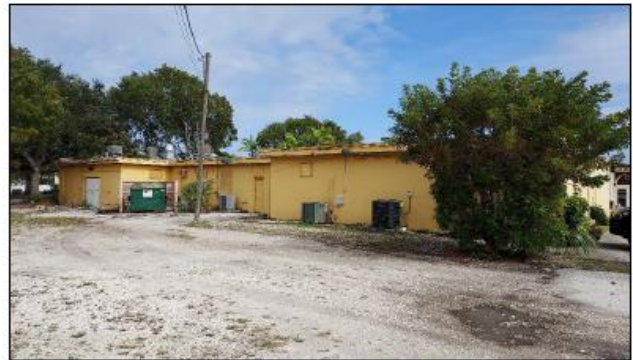
VIEW OF REAR OF SUBJECT BUILDING
