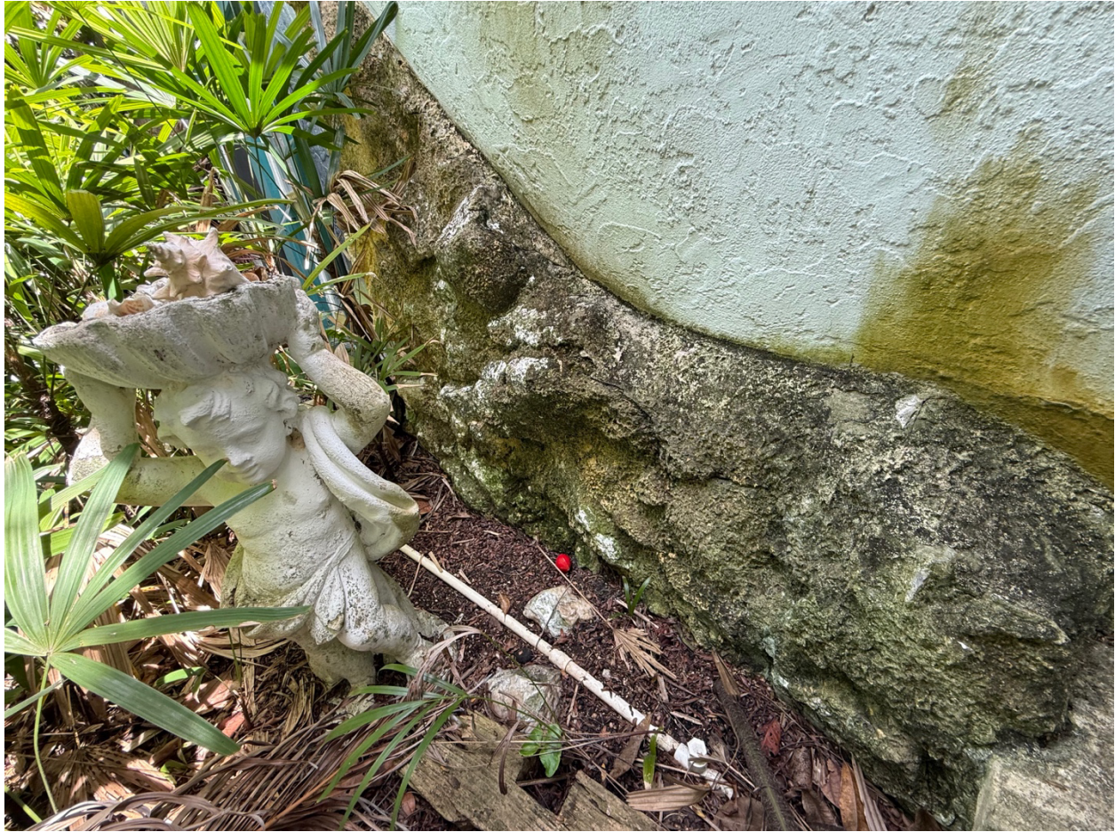
Current Existing Coral on North Elevation
