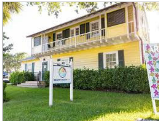
20 N Swinton Ave – CRA Office
