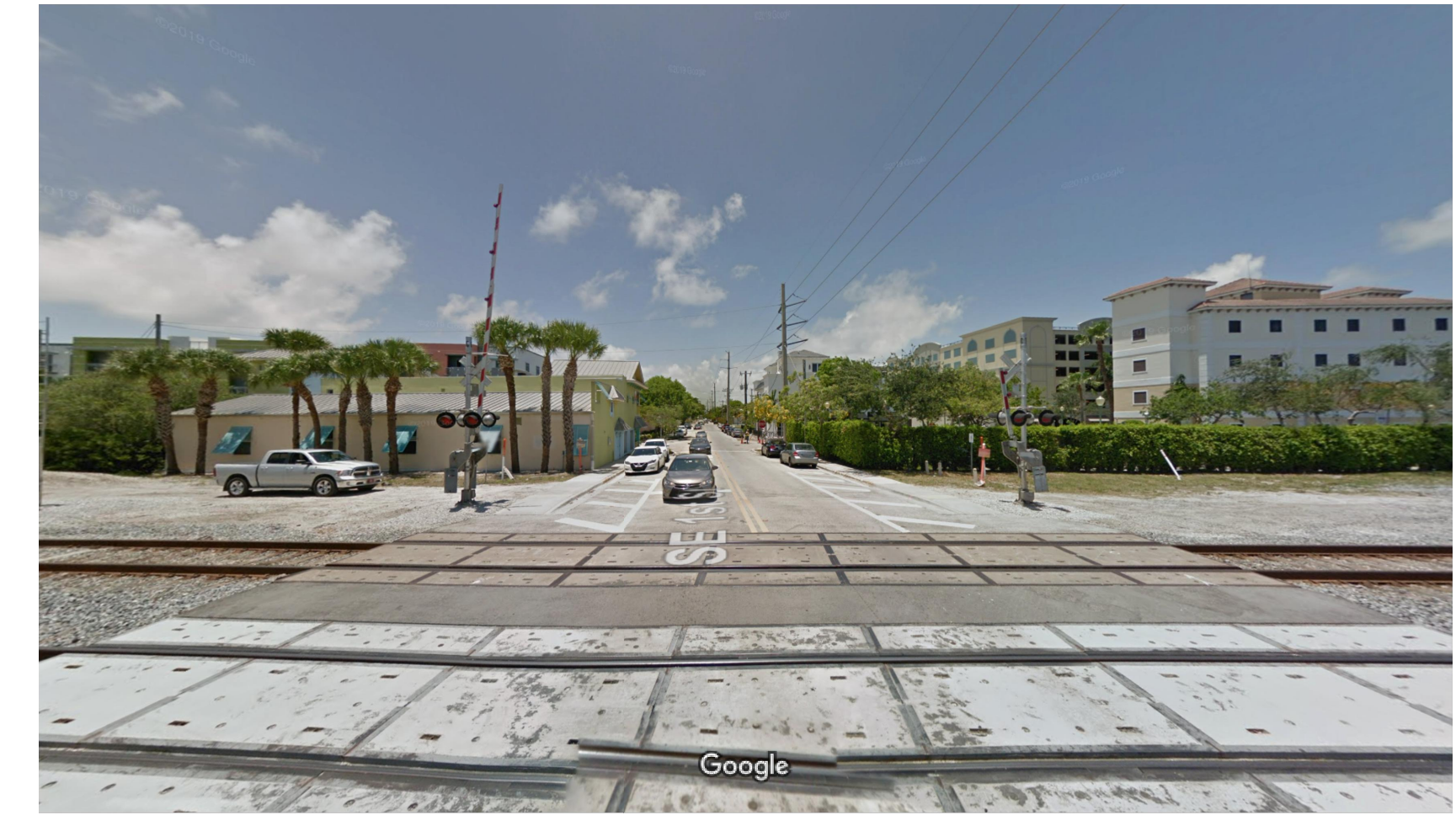
6 East view of Site along SE 1st Street/FEC
