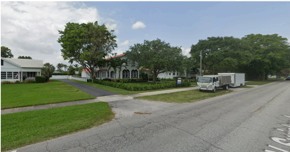
South view of exiting House from R.O.W.
