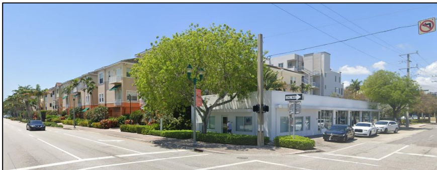
Adjacent property to the southwest corner
