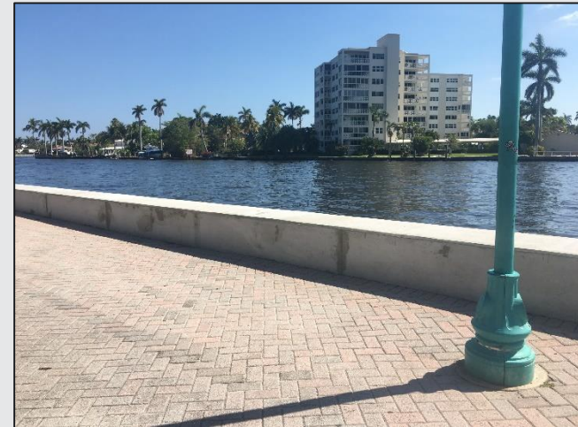
2018 Veteran's Park Seawall Improvement
