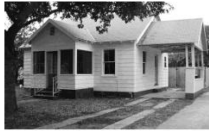
An example of weatherboard siding
