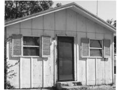
Board and batten siding
