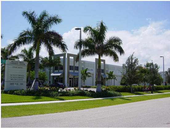
Wallace Drive Office/Warehouse, Delray Beach
