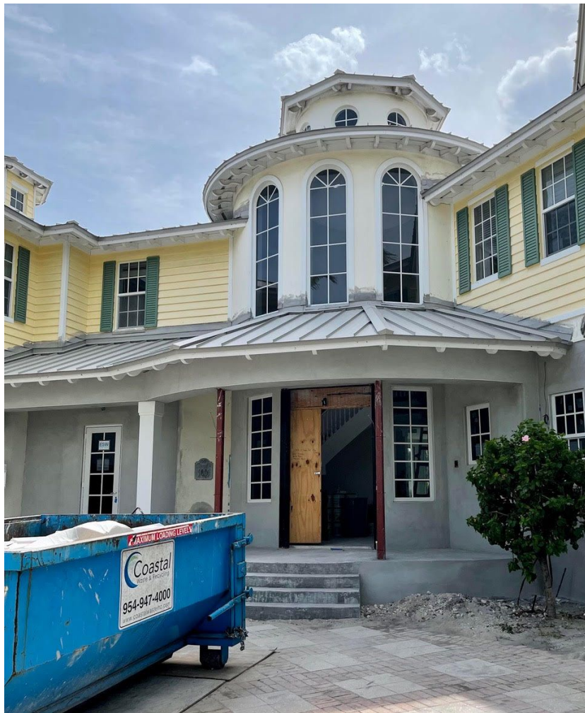
1001 N VISTA DEL MAR RAISE EXISTING FINISH FLOOR TO MEET 7' CODE
