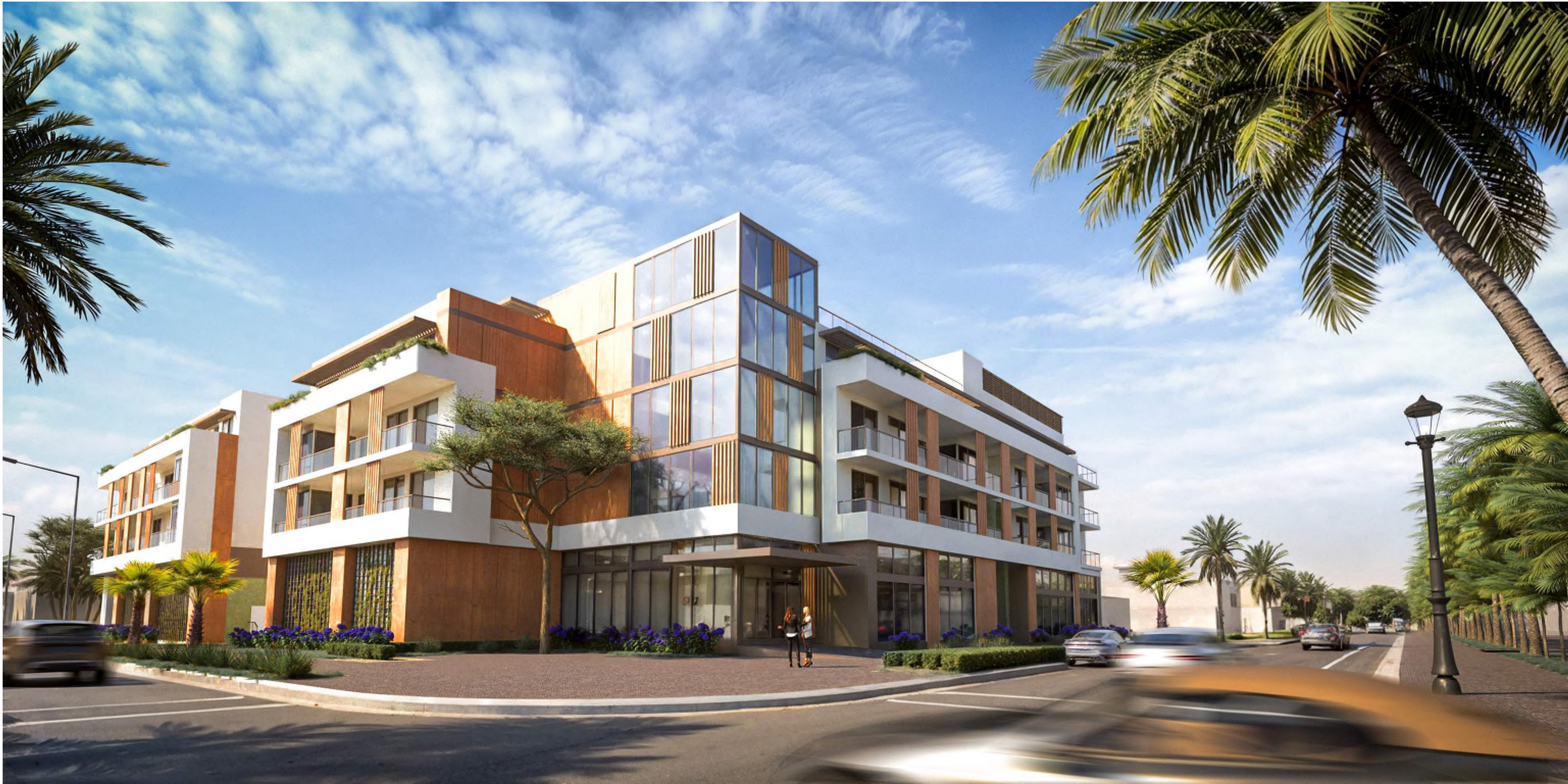
NORTH - WEST CORNER
