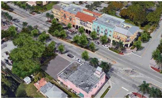
Existing West Atlantic Avenue
