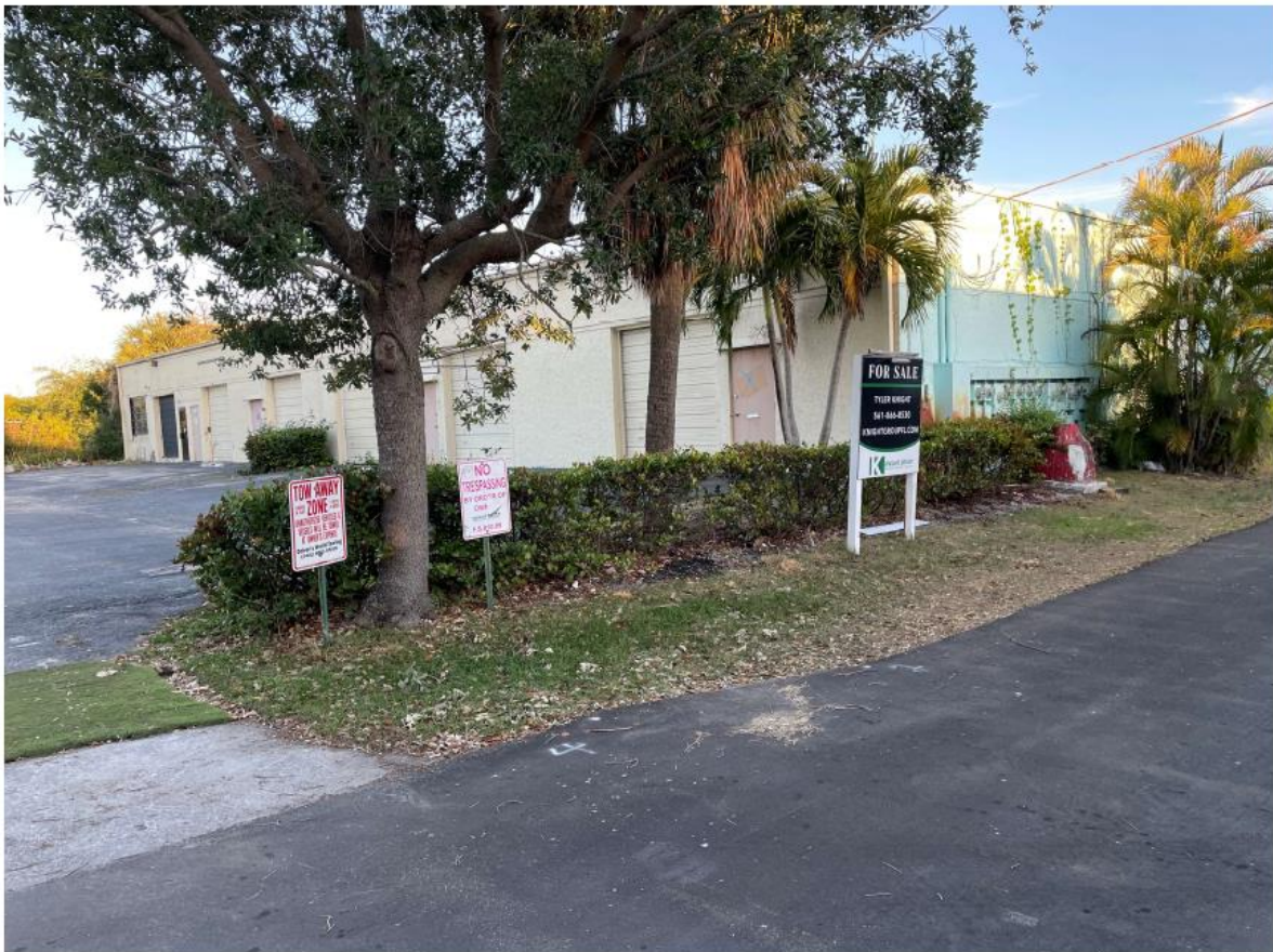
Facing subject 350 building from Artists Alley (north and west elevations shown)
