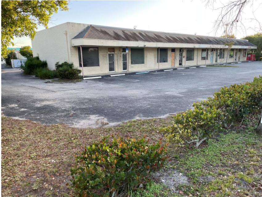
Facing subject 330 building from NE 4 th St (east and north elevations shown)
