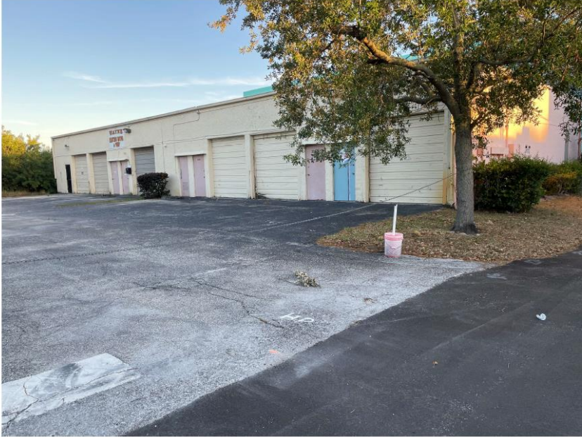
Facing subject 358 building from Artists Alley (north and west elevations shown)
