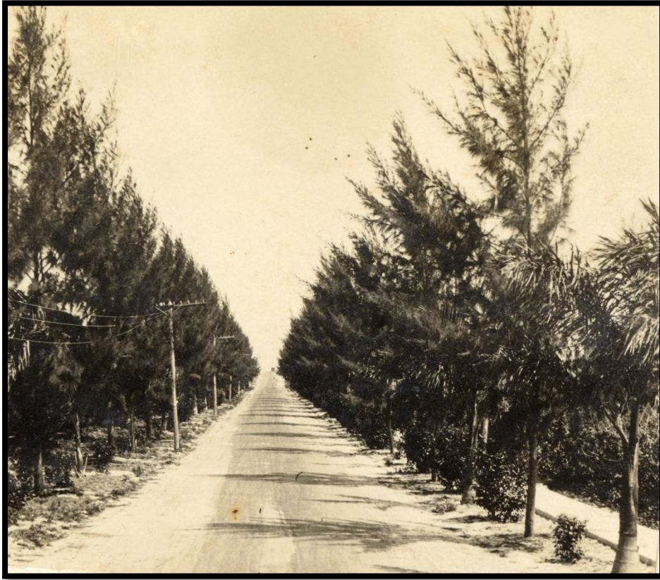
FIGURE 13. East Atlantic Avenue, circa early 1920s. Notice the early power lines on the left.
