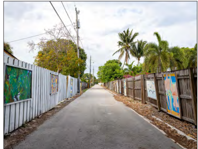
Figure 11 Infrastructure Project – Osceola Park Neighborhood Improvements
