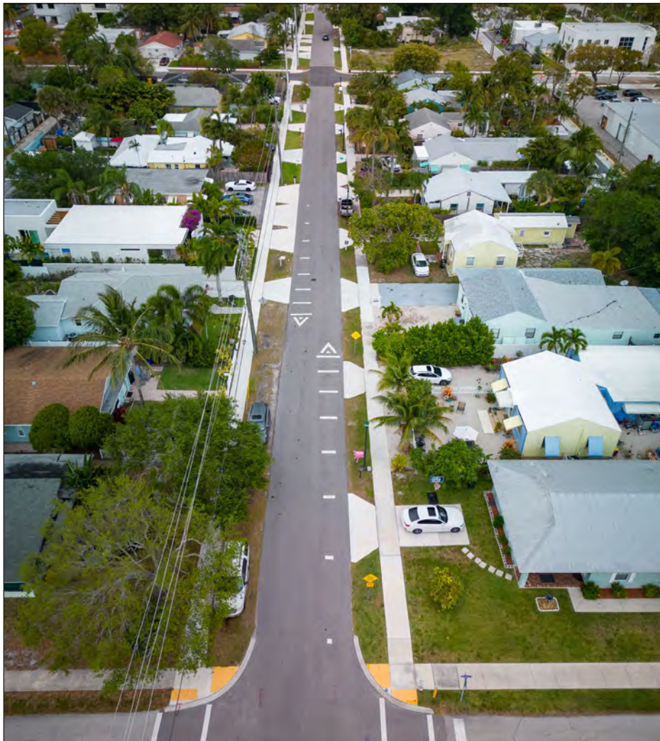
Figure 10 Infrastructure Project – Osceola Park Neighborhood Improvements
