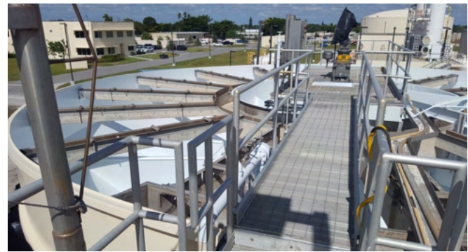
City of Sunrise - Springtree Water Treatment Plant Ion Exchange System Improvements. Carollo provided renewal and replacement of the 24-mgd lime softening facility, which included design of a fluidized-bed IX treatment system. The IX system will reduce TOC, control color, and minimize DBP formation potential.
