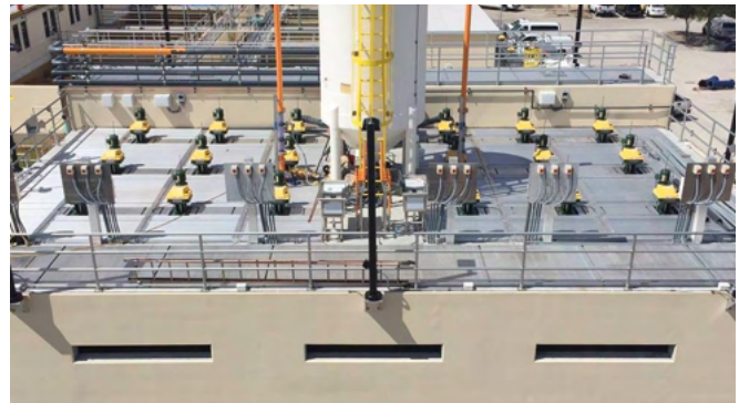
City of Boynton Beach - IX Plant and East WTP Improvements. Carollo designed and constructed a 16-mgd MIEX treatment process to pretreat water from multiple wells prior to the lime softening process.
