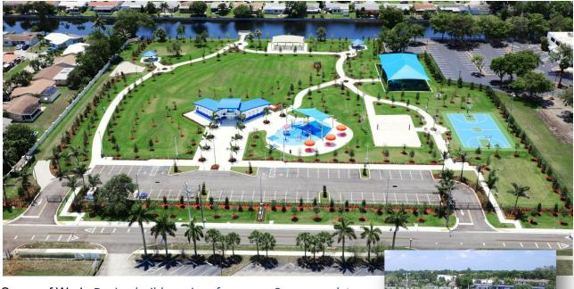
Scope of Work: Design build services for a new 6 acres park to include 1,000 SF restroom/storage/IT room building, 9' wide concrete walk, 9 exercise ADA stations in covered area, full size basketball court NFHS compliant w/ asphalt, base and acrylic surface, Sand Volleyball court, (2) 24' Hexagonal shelters, 3,000 SF splash pad, 4,000 SF playground, site furnishings, fishing pier, parking, fencing, lighting, landscape, irrigation, WIFI/security.
