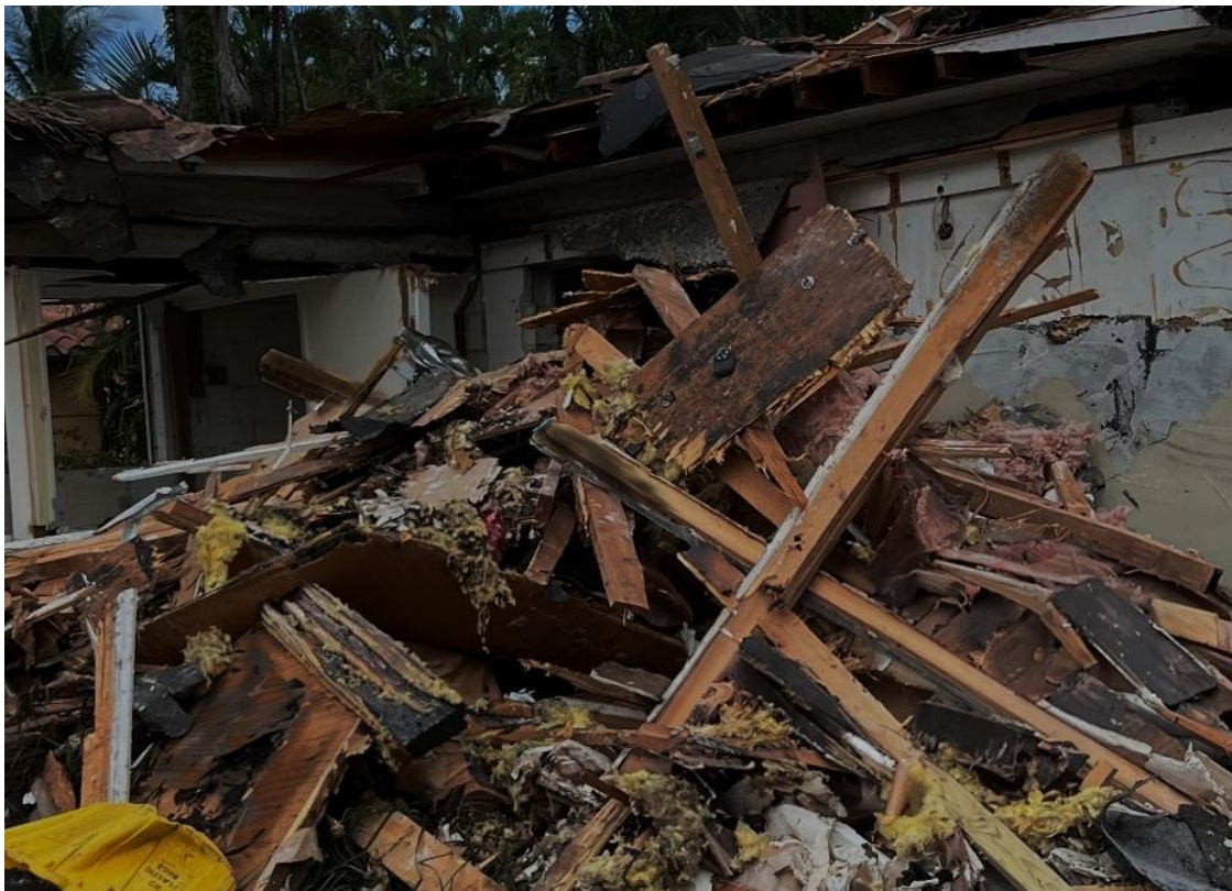
Rotted, defective wood removed
