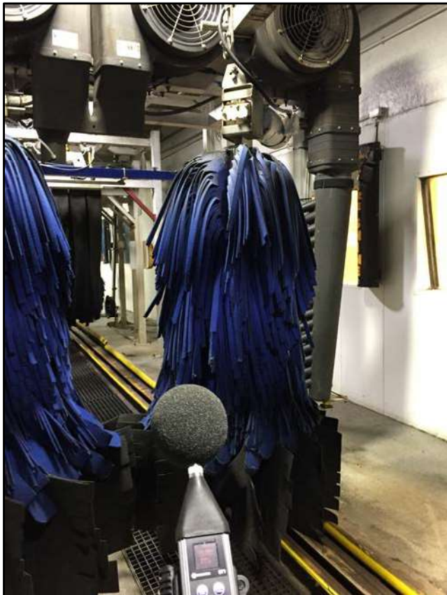
Photo 3. Dryer Blowers Without Silencers
