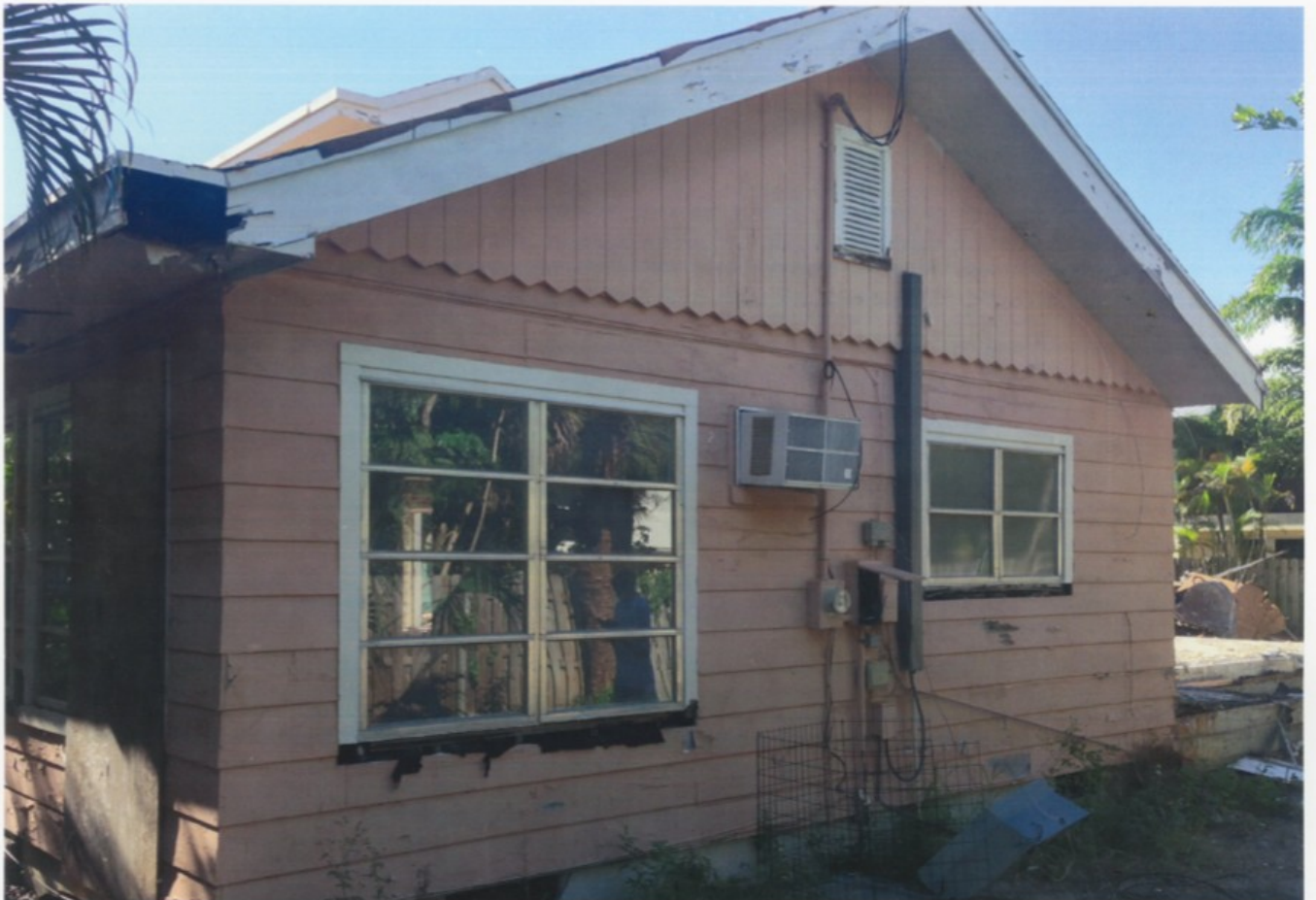
55 SE 7th Avenue-Original East Exterior-August 2014
