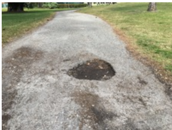
Typical asphalt cart path with pot hole.
