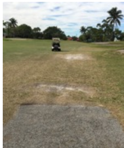
Noncontinuous cart paths have created difficult conditions to grow turf due to compaction, wear and tear.
