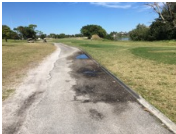
Asphalt cart path with worn edges, pot holes and holding water.
