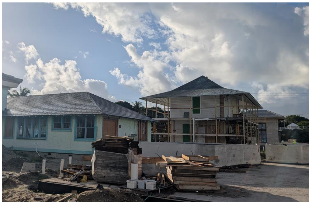
Buildings C and E-The Cathcart House existing on site.
