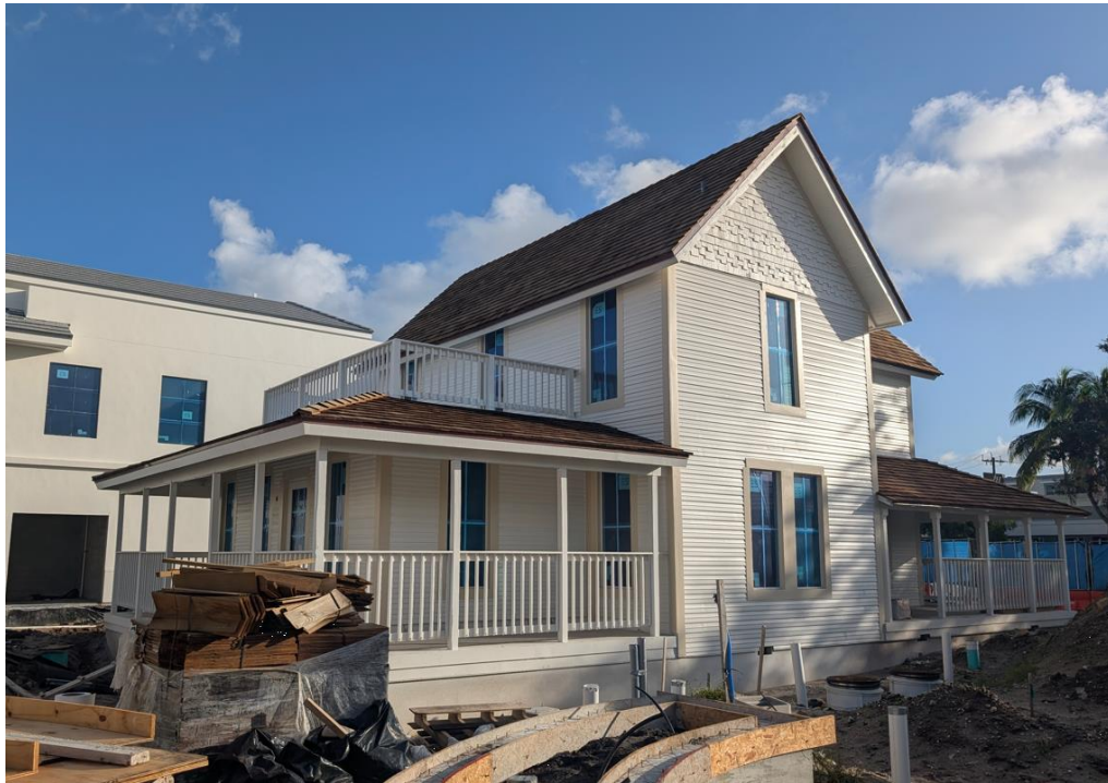
Siding was repaired and replaced on Building A- The Rectory
