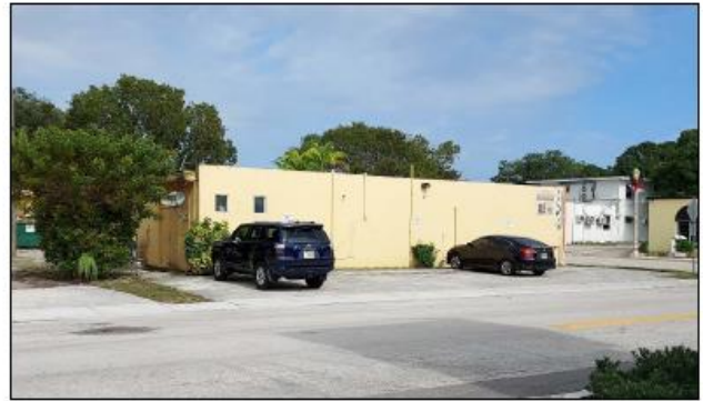
VIEW NORTHEAST OF THE SUBJECT FROM NW 1ST STREET
