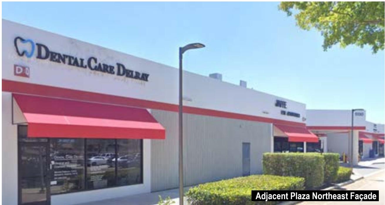
Adjacent Plaza North Façade
