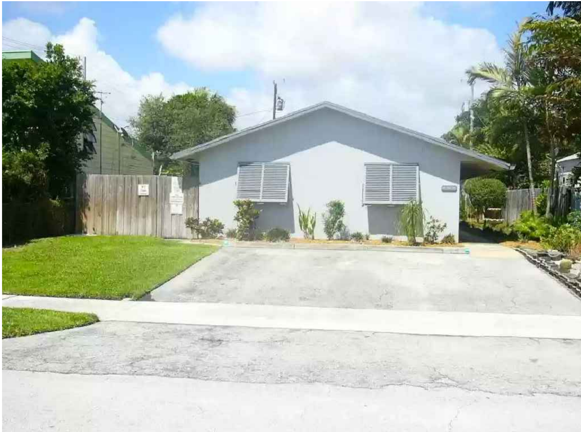
EAST ELEVATION-304 NE 1ST AVE
