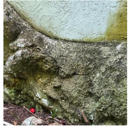
Existing Coral Feature (North Elevation)
