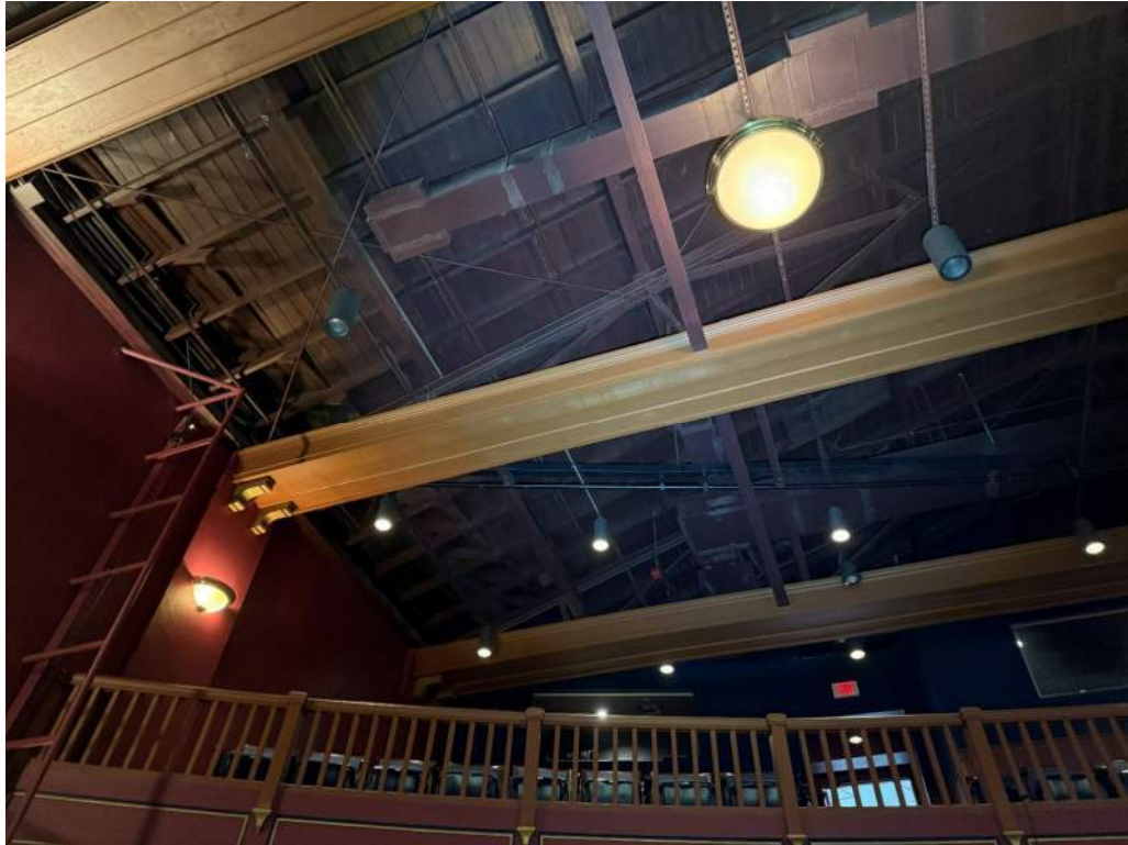
Photograph 1 - Steel Trusses in Auditorium
