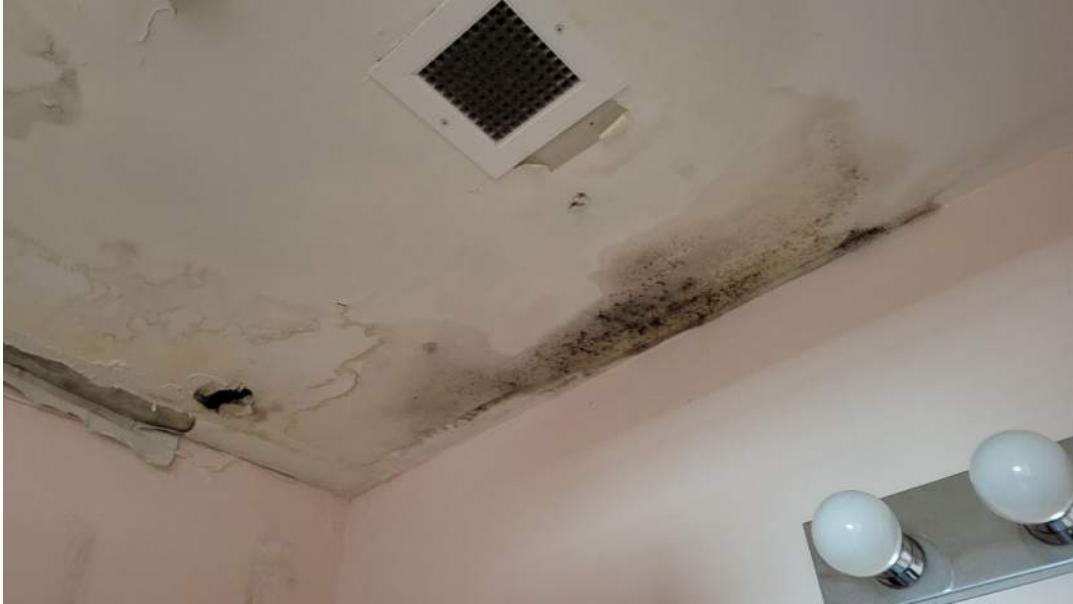
Figure 26. View of moldy shower ceiling in second floor toilet room.
