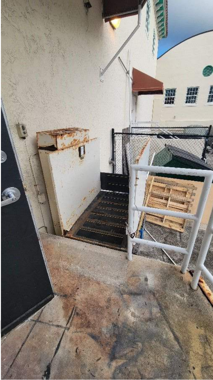
Figure 21. The existing lift at the loading dock is in poor condition.
